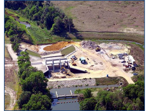
NEW CONSTRUCTION OF THE P-11 STRUCTURE
