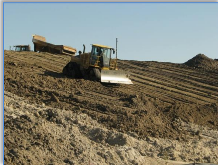
GPS Controlled Dozers Grade the Slope
