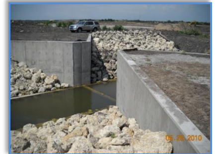
Weir and Stilling Basins
